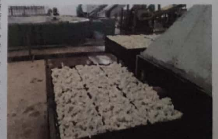
Figure 2 Rubber lump production plant (RPGL)
